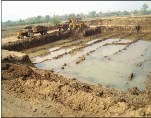
Rain/ runoff water storage structures developed in the tail-end (Madhyamkhanda sub-minor)
