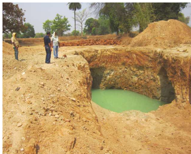
Dugwell under construction at the project site
