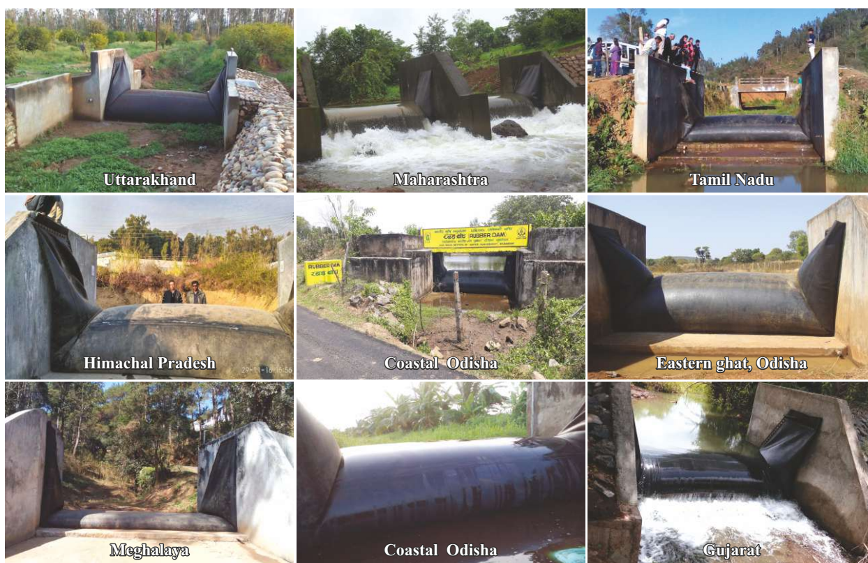
ICAR Flexi-check dams installed in different agro-ecological regions of the country
