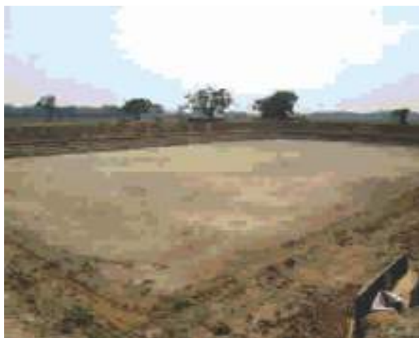
Tank-cum-well system of 80 m length, 60 m width and 2 m depth, with a harvested volume of 10,000 \text{ m}^3 during the monsoon season of 2014
