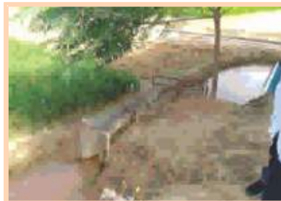
Parshall flume installed for measurement of irrigation water
