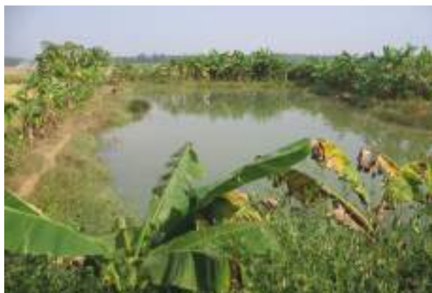
Water storage tank under Soroda sub-minor (II)
