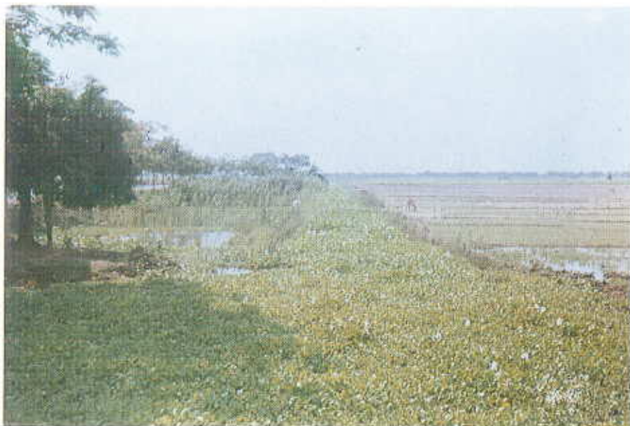
Infestation of water hyacinth causing reduction in carrying capacity of open drain
