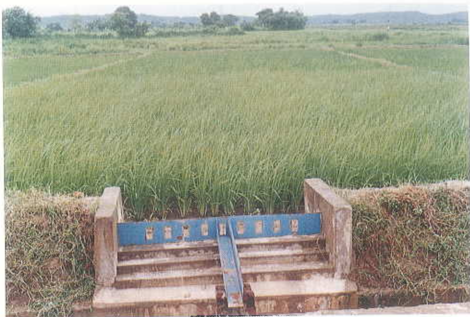
Experimental field with multislot divisor.
