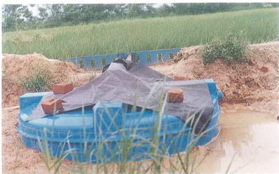
Fibreglass rainfall excess collection tank.
