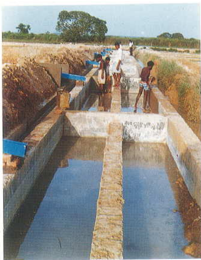
Brick masonry rainfall excess collection tanks.
