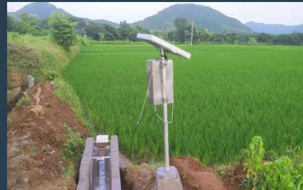
Device installed in farmers' fields
